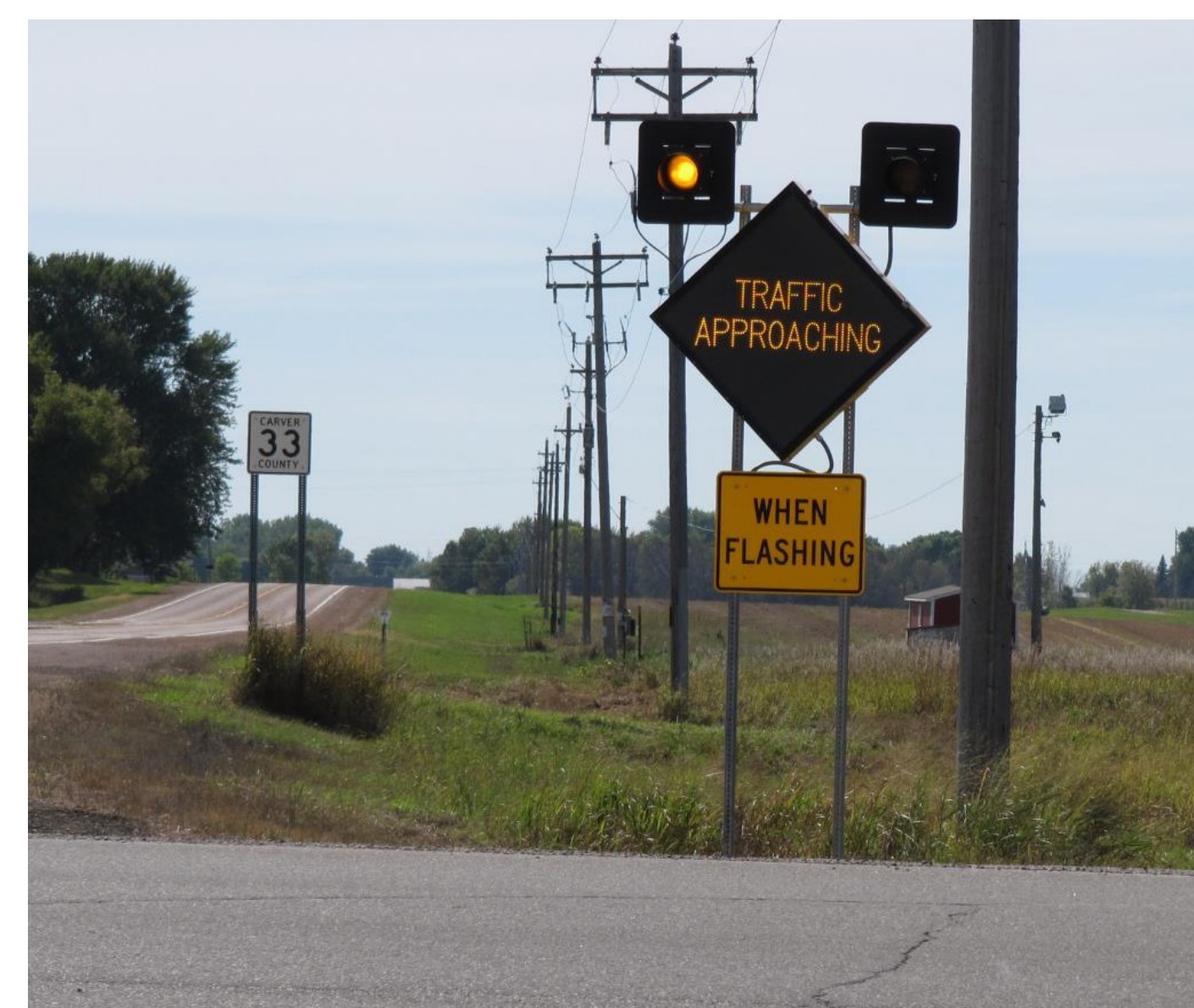
Rural Intersection Conflict Warning System (RICWS)
